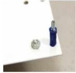
Screws instead of rivets allow easy upgrade or replacement
